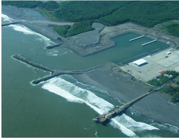
Photo 4: The old pier and the new port, May 2010
