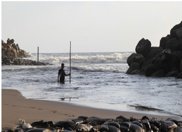
Photo 8: Only small fishing boats can enter the access channel due to its limited depth
